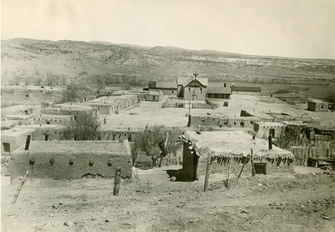
Plaza, Abiquiu, New Mexico, ca. 1915-1920? Photographer: T. Harmon Parkhurst, Negative Number: 013698. Courtesy Palace of the Governors Photo Archives. The house O'Keeffe purchased is behind the church on the far side of the plaza. The village looked very much like this when Maria began construction on the Chavez house.
